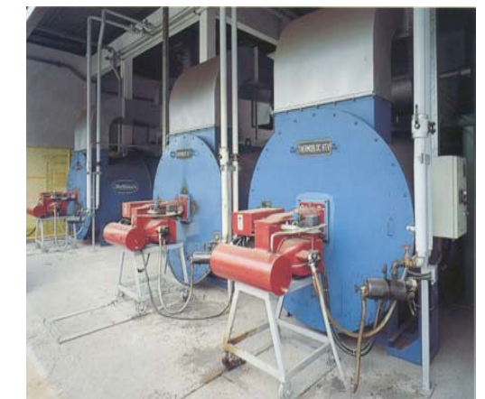
INDIRECT gas or oil fired air heaters for medium and high temperatures.
